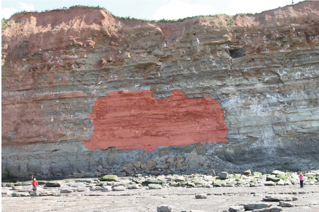
Figure 4: Photograph (14/04/13) showing the location and extent of the rockfall observed between 14 th March and 14 th April, with debris pile below. Note people for scale.
